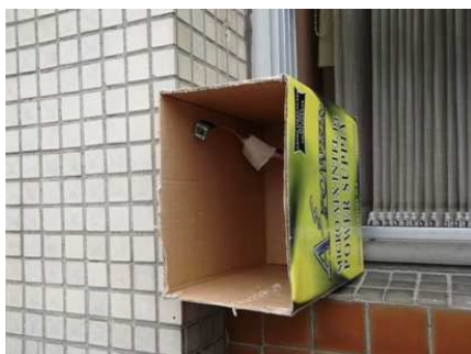
Fig. 5. Outdoor sensor installation
